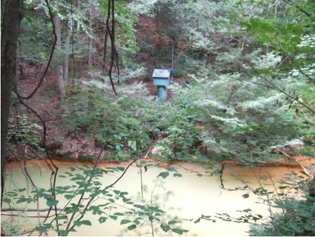
PHOTO 11: LOOKING AT LEFT BANK AT TUNNEL OUTLET
