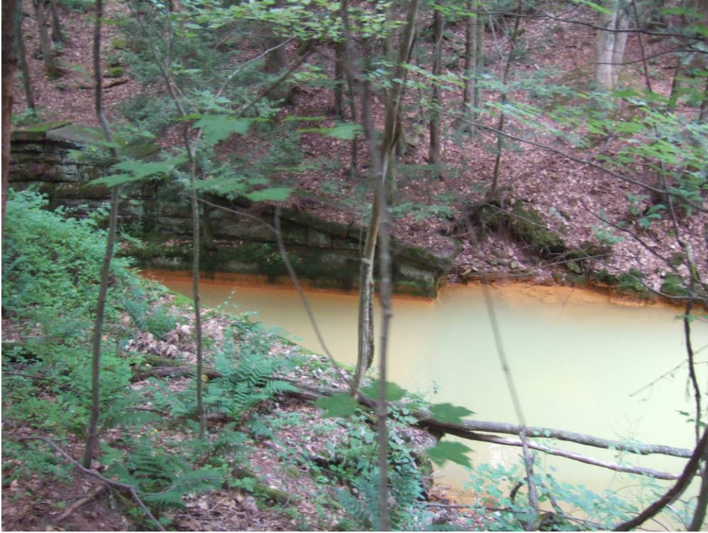
PHOTO 7: TUNNEL OUTLET FROM RIGHT BANK
