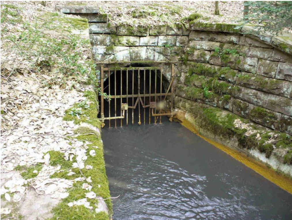
PHOTO 6: JEDDO TUNNEL OUTLET
