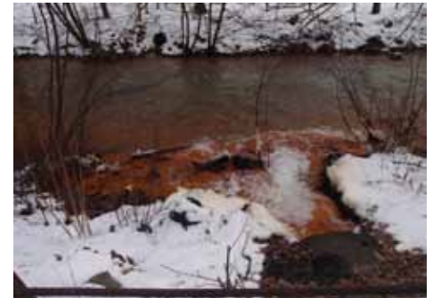
The Oakland Tunnel entry to Mahanoy Creek.
