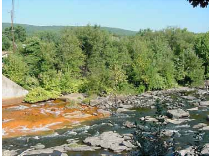
The Old Forge Borehole from the western bank of the Lackawanna River.
