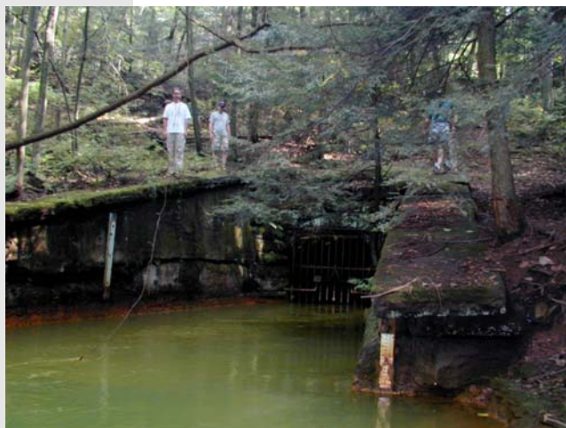
Image 1.21 The Jeddo Tunnel (source: Project Team)
