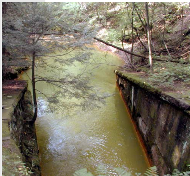
Image 3.9 Jeddo tunnel outfall (Source: Project Team).
