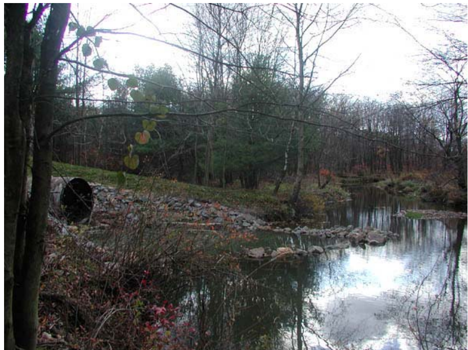
Image 3.3 Stormwater overflow into Black Creek in Hazle Township (Source: Project Team).
