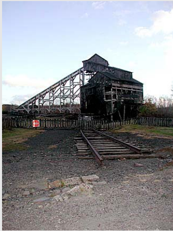
Coal Breaker at Eckley Miners' Village. (Source: Project Team)
